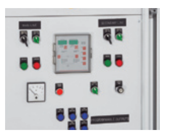
Control panel of a supply inverter
