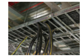
Swifts cable ladder: main distribution infrastructure
