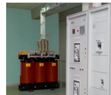
Zucchini transformer and busbars, XL³ enclosure with DMX³ supply inverter
